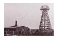
The most prestigious project of Tesla was the Wardenclyffe Tower, located in Shoreham in the USA state of New York. Its purpose was to transmit wireless electricity, together with all sorts of wireless communication (including telephony). The picture to
